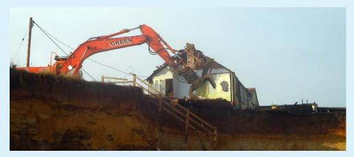
Figure 13: A property at risk of coastal erosion being demolished (image courtesy of North Norfolk District Council).
